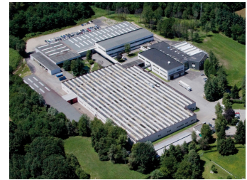
Sesto Calende plant
